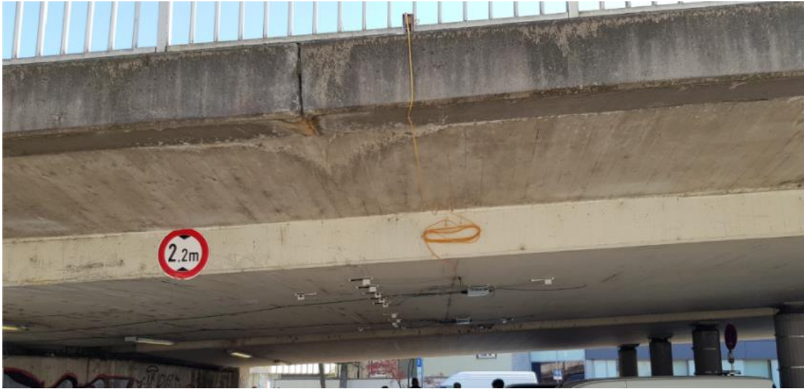
Figure 8.5. Position of spiders on the slab (Cervenka et al., 2020(b)).
